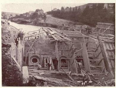
WO views looking up stream showing the forms for waste way near the eastern bank. In No. I you will notice that there is a rabbet in the buttresses to receive a floor over the waste way, in order that when the gates are open the waste water can not interfere with the passage-way through the dam, which is seen above the floor level.
